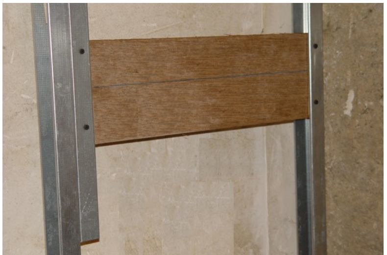
afb. 18 - 11 Achterhout -> multiplex placed for heavy loads
