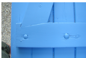
afb. 09.4.5 - 7 don't make a brace like this ...
