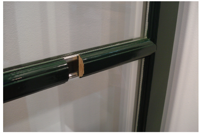
afb.9.2.3 - 2 Aluminium ingetroedes achter de opgeplakte sporten. -> Aluminium profiles in between the double glass, behind the wooden bars.
