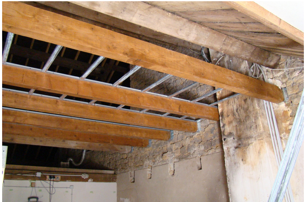
afb.08.3.4 - 10 Rails aan bovenkant balk -&gt; L-profiles near the upper part of the beams
