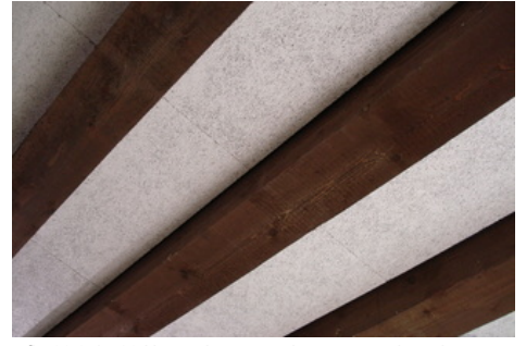
afb. 08.3.4 - 22 Houtwol-cement-platen -> wood-wool-cement boards - don't like it
