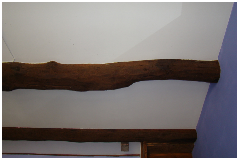
afb. 08.3 - 20 gipsplaten tussen kromme balken -> plasterboard placed between irregular beams
