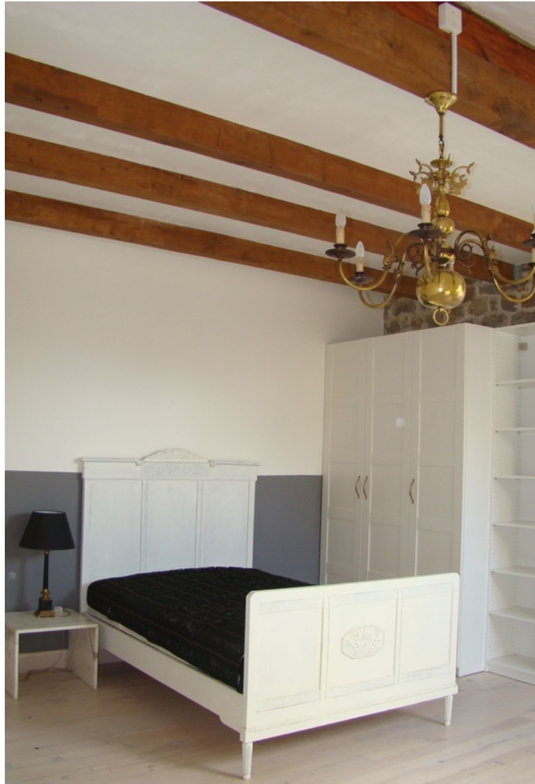
afb.08.3 - 19 gipsplaten tussen balken (hier relatief rechte) -> the plasterboards between the beams (these are relatively straight)
