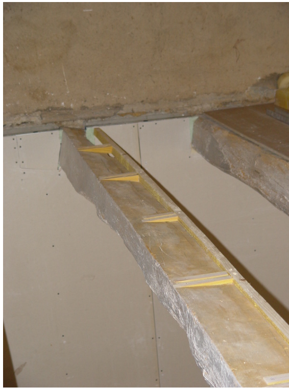
afb. 08.1.4 - 12 Deze balk is echt sterk getordeerd! -> A strongly twisted beam made flat with a batten and a series of wedges.
