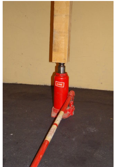
afb. 08.1.4 - 4 balken opkrikken -&gt; lift a beam with a bottle jack
