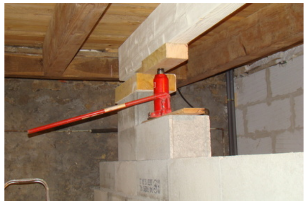
afb.08.1.2 - 8b 8ton-potkrik onder de balk -> bottle jack under the beam
