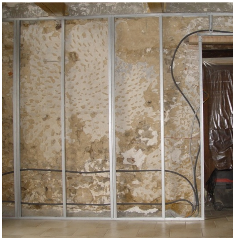
afb. 07.1.1 - 18 Flex-buizen (gains) ingereggen in de gaten van de staanders -> gains for electric cables placed in the openings of the studs
