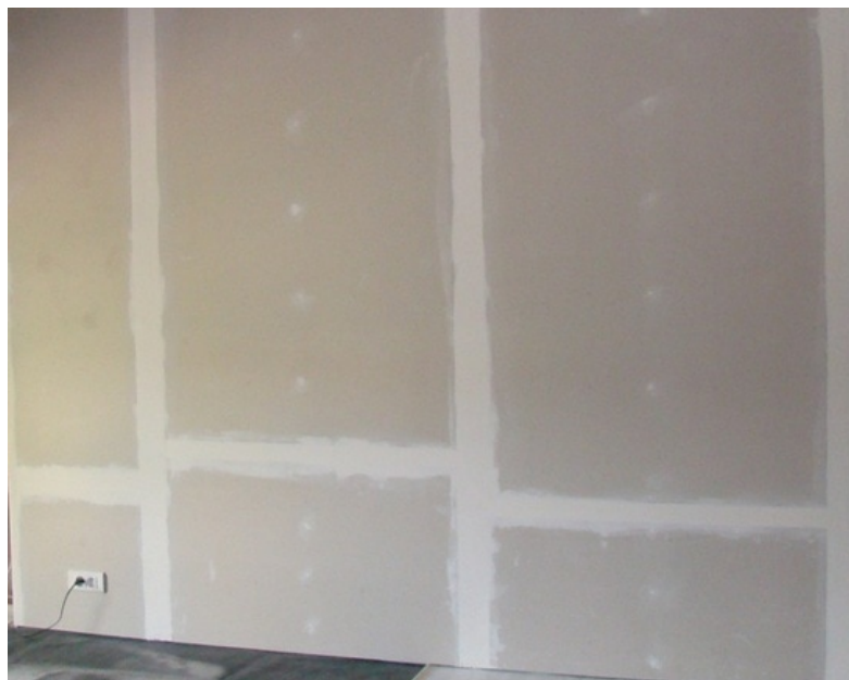
afb. 07.1.1- 33 Verticale naden met papierband afgewerkt, horizontale naden V-vormig uitgesneden -> vertical joints (tapered edges) finished with paper tape and filler, horizontal joints with deep V-joints just filled with jointing compound. The room was 2,70m high.
