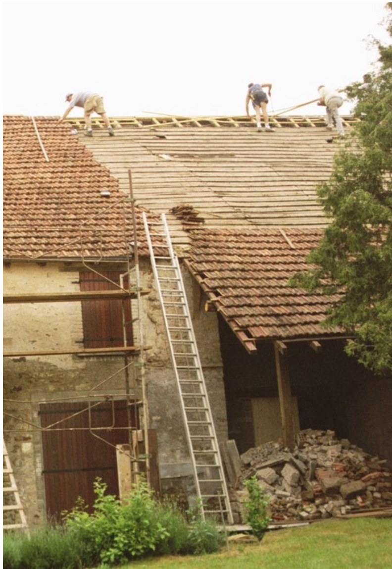
afb. 06.3 - 1 -&gt; removing the tiles and the old battens
